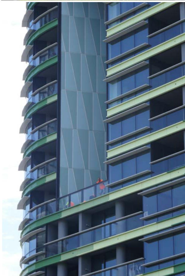
Figure 2. Close-up view of a 6 storey slot. Note the 6 panels forming the load bearing wall of the inset slot, each one storey high.
